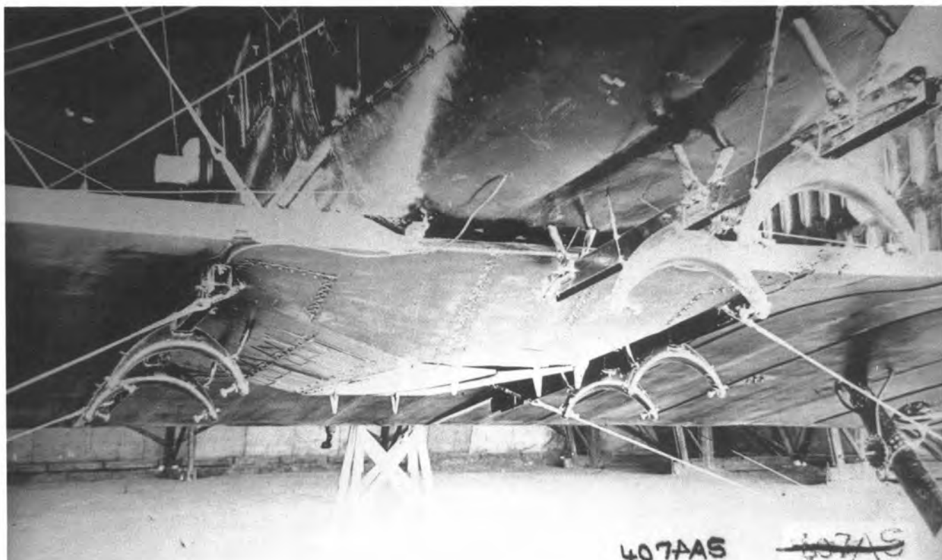
Close up view of the torpedo racks on a Caproni Ca.3 (Ca.33). This type was a forerunner of the Ca.5 which the Northern Bombing Group planned to use when operating with 214 Sqn RAF. :1361st AV Sqn via Noel Shirley
