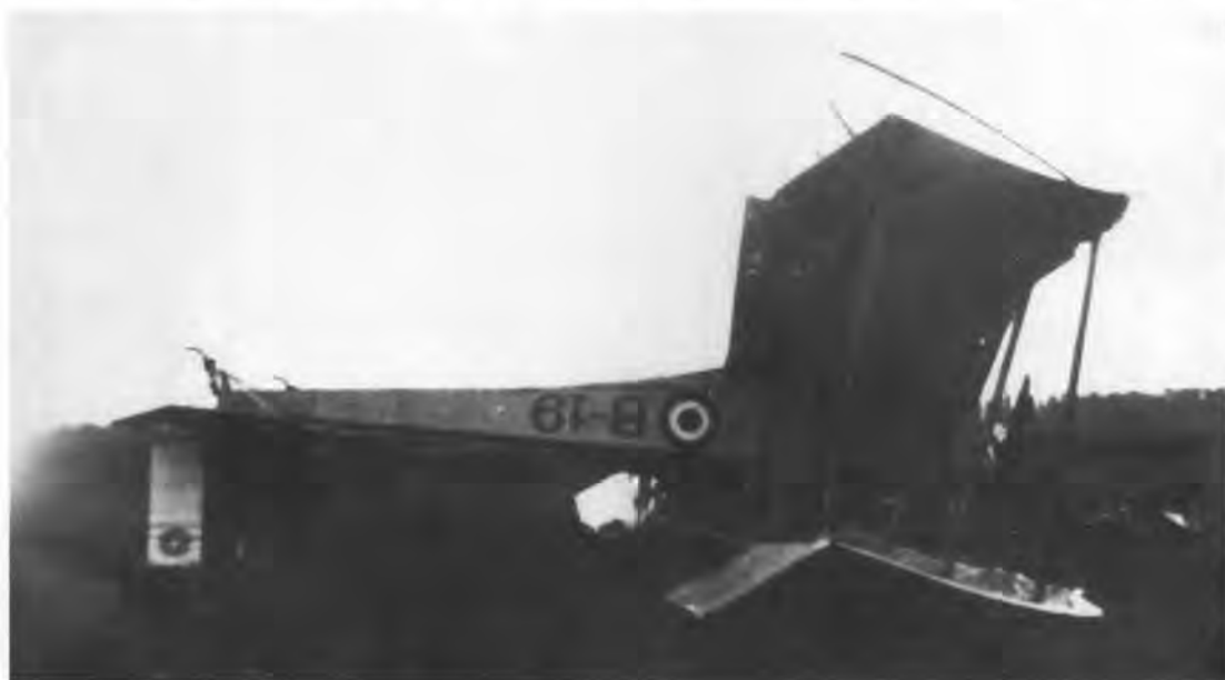
Caproni Ca.5 (Ca.44) B-19 of the Northern Bombing Group. This machine crashed at Dijon on 2 September 1918 on its delivery flight from Milan. Ex-Italian serial 11589; a small USAS cockade is painted on the left rudder. :C.D. Dushane via Noel Shirley
