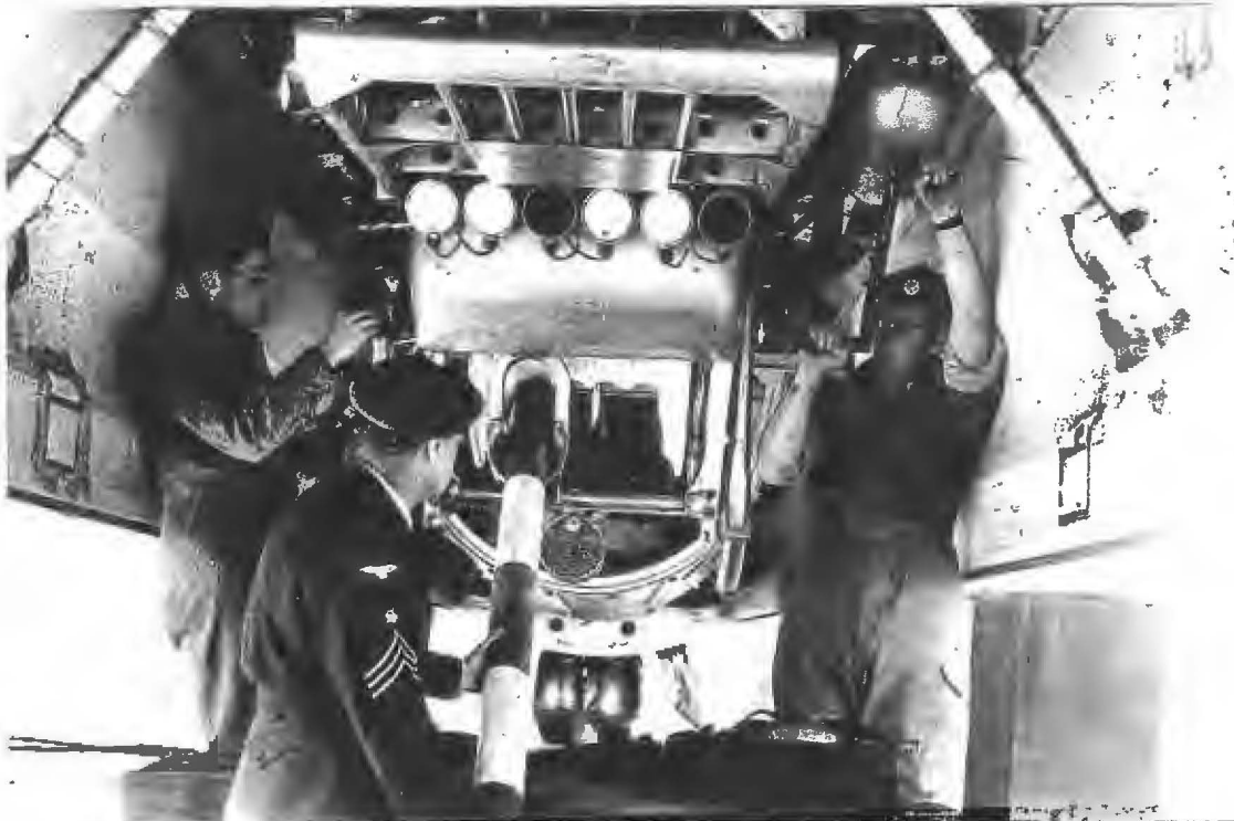
Hose Drum Unit (HDU) installed in the bomb bay; winding in the hose.
